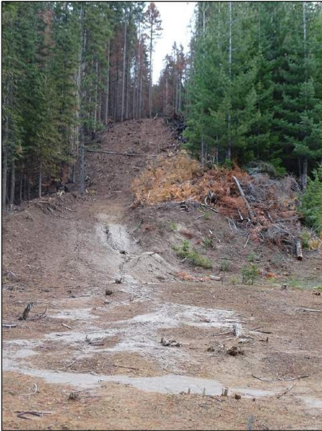
3(c)i Erosion from a steep dozerline Johnson Creek Fire, Idaho 2017. Photo credit: Friends of the Clearwater
